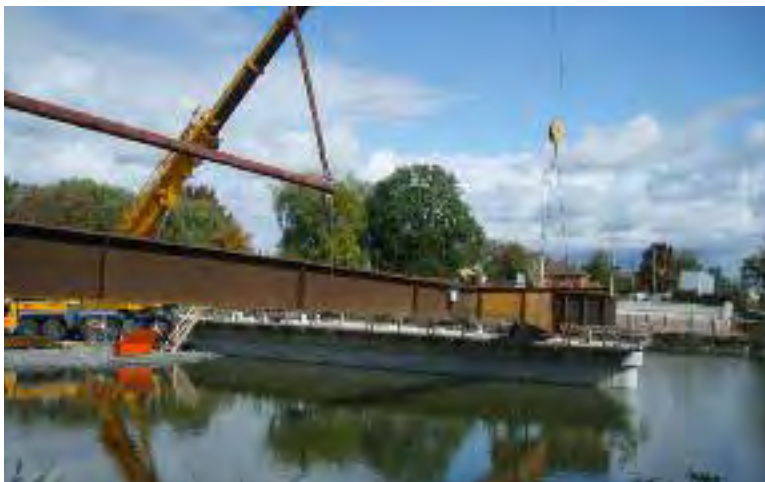
Construction of the Veteran's Memorial Bridge
