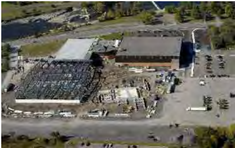
Construction of the Belleville Multiplex Recreation Community Centre
