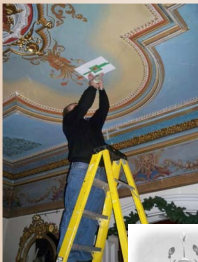
(above) Testing the paint surface of the South drawing room ceiling.
