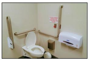
Photo Five: A fully renovated washroom with accessible features such as grab bars, toilet and toilet paper height placement, and an audible and visual emergency push button.
