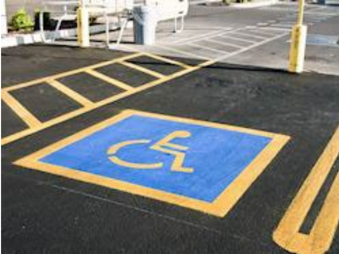
Figure 4: Example of pavement marking used to identify a designated accessible parking spot
