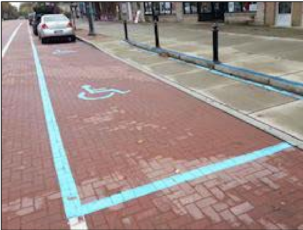
Figure 10: An example of on-street designated accessible parking where there are access aisle spaces on both sides and the front and back of the spot. (source: gaates.org/DOPS)
