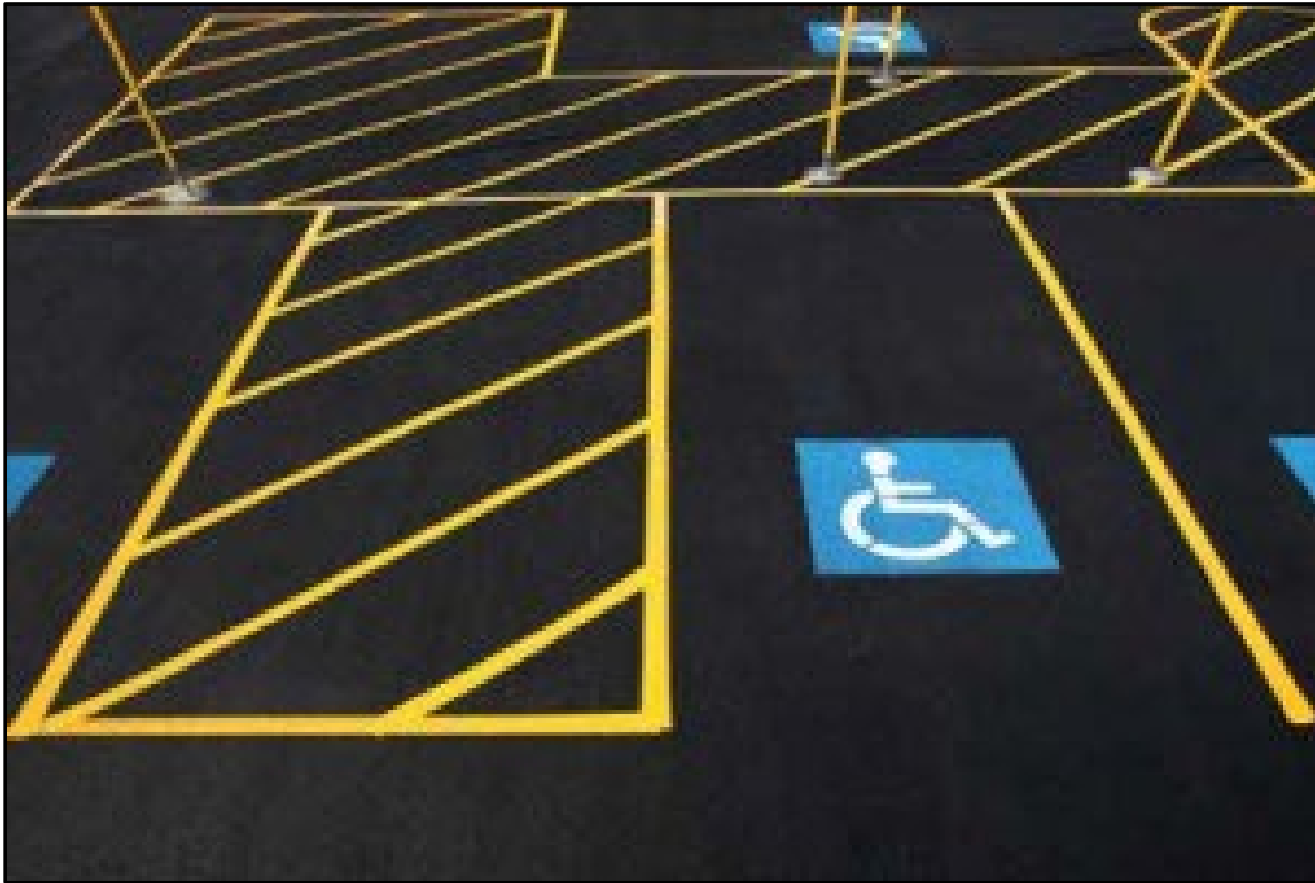
Figure 9: An on-grade path of travel route delineated with yellow horizontal pavement markings provides clear indication of a safe and accessible route from designated accessible parking spots to the nearest sidewalk or building entrance.
