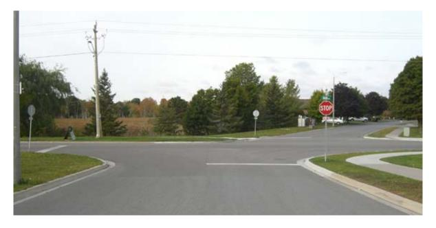
The Victoria/Haig Intersection is a two-way stop-controlled intersection with Haig Road forming the north-south approaches and Victoria Avenue the east-west approaches. The following shows the lane configuration of the intersection:
