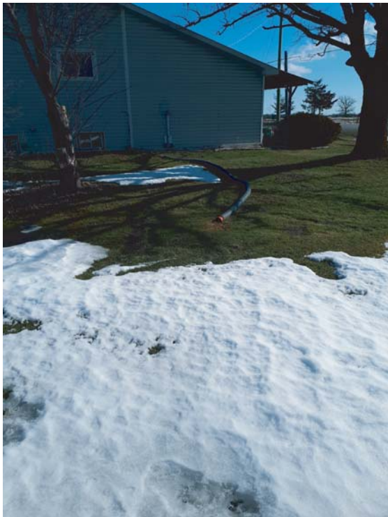
Photo C (above): Sump outfall
