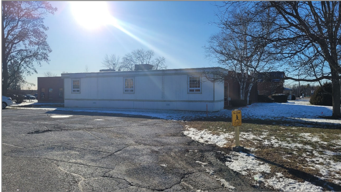
Looking west at existing office trailer on the subject property.
