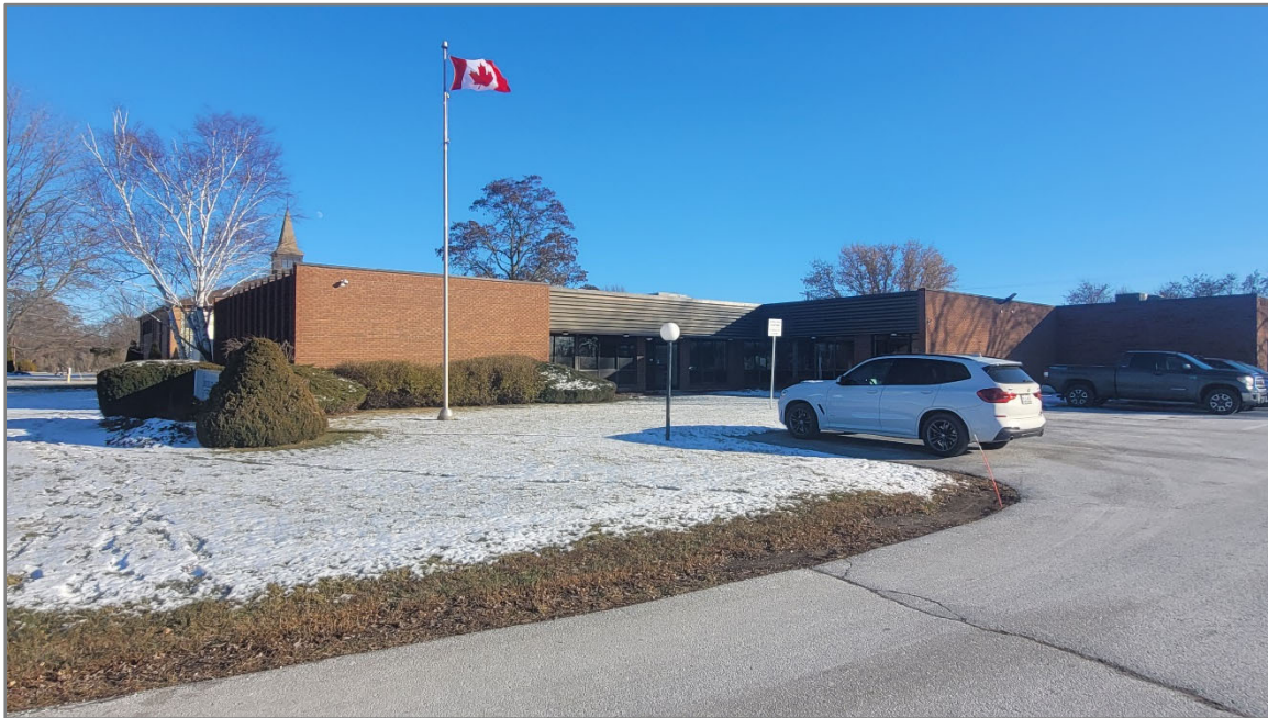
Looking at front of existing office building on the subject property.
