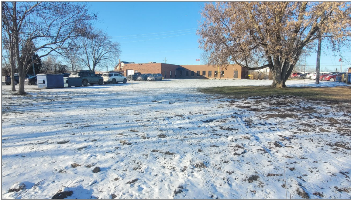
Looking north at existing office building on subject property.
