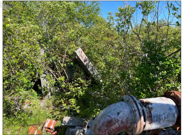
Photo 12—Rubble north of the pump house looking north. May 26, 2023.
