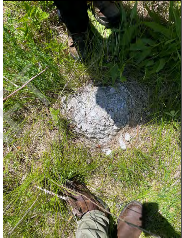
Photo 14 – Potential decommissioned well near BH05. May 26, 2023
