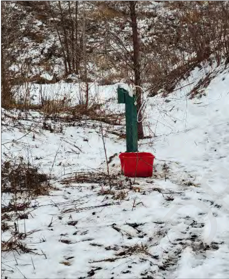
Photo 7 – MW215 looking south, installed December 2022.
