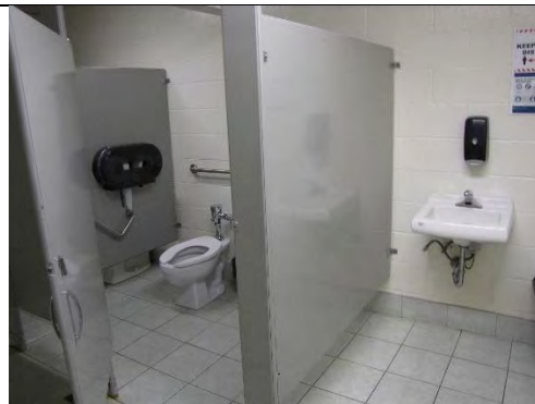
Toilet stalls do not have a 1500 mm turning radius
