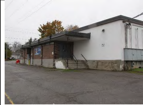
Exterior brick and stucco on the main community building
