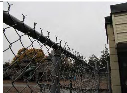
The chain link fence abutting the building allows for climbing access to the roof, allowing for the possibility of vandalism. It also is a liability risk.
